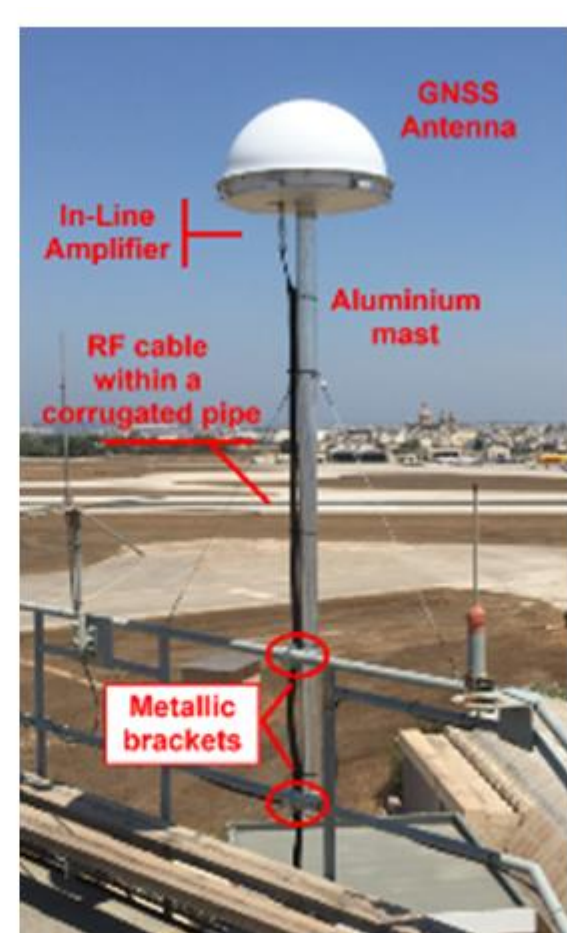
(b) Installation of the GNSS antenna on the tower of Malta airport (with a sketch of the coax-cable path)
